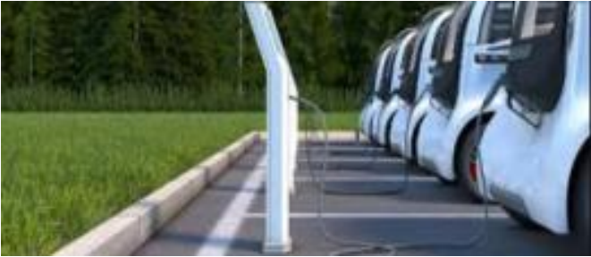
Building infrastructure to accommodate 10 million EVs (Source: SSE)
